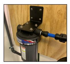
Be sure to use fasteners compatible with the wall material. The filter needs to be secured to studs or a backing board. It will be very heavy once it is filled with water.
