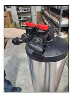
12. Prepare the filter housing by installing the bracket on the housing and tightening the screws. Be sure to use the supplied washers. The filter should flow **left to right**. Install the threaded quick connect fittings in the filter housing. Be sure to use Teflon tape.
