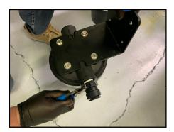
13. Install PEX tubing in the outlet fitting previously installed on the filter sump. This will connect to the "Upflow" Inlet on the tank.
