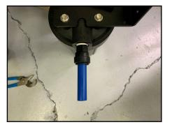
14. Level the filter housing and make sure the pipe is not in a bind then install wall fasteners (not included) to secure the filter housing to the wall.
