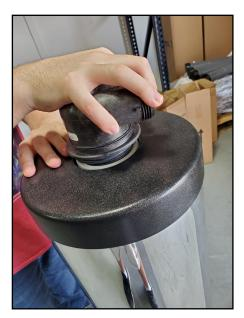
9. Place the Bodyguard Whole House Chemical Removal Filter tank in the desired location. Typically this is at the water inlet of the home.
