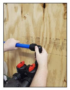
13. Place a bucket under the outlet port (Upflow Inlet) of the Fluoride tank or run a line from the outlet port of the tank to a drain. Place the bypass in the service position.
