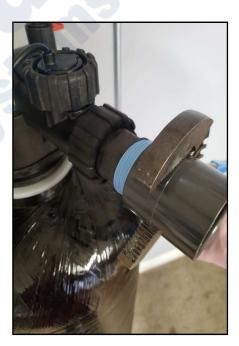
NOTE: All piping should be secured to prevent stress.
