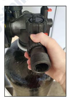
5. A three valve bypass should be installed in the plumbing for service purposes.
