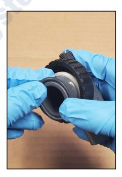
10. Lubricate the O-rings on the supplied bypass with the silicone grease. Install the bypass on the tank and fully tighten the retaining nuts. The bypass will move slightly once tight. It is made to flex and move and will not be rigid. Be sure the O-rings are lubricated on the elbow connectors previously assembled. Install the elbows in the bypass valve and tighten the retaining nuts. These will move when tight. They are made to flex just like the bypass valve connections.
