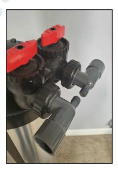
11. Connect the cold water supply to the "Up Flow" inlet of the Upflow Calcite pH Neutralizer Filter tank
